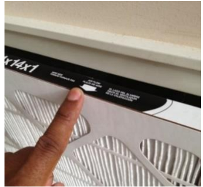
Changing pre-filters regularly extends life of HEPA filters.
